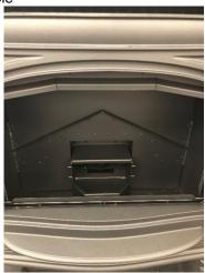
8. With the liners removed, clean all fly ash and debris from the firebox. Clean the liners before replacing. Make sure to clean the heat exchanger on the firebox ceiling.
